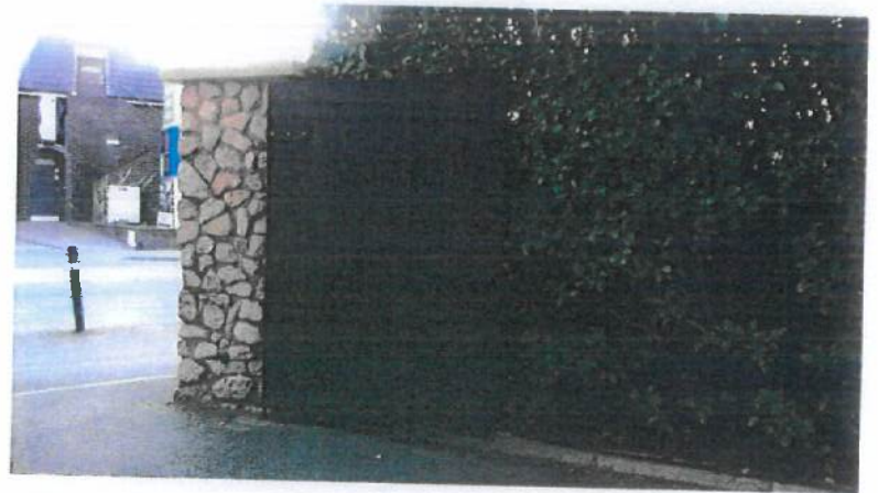
Open Gate with Granite Capping Stone on Granite Random Rubble Pillar
